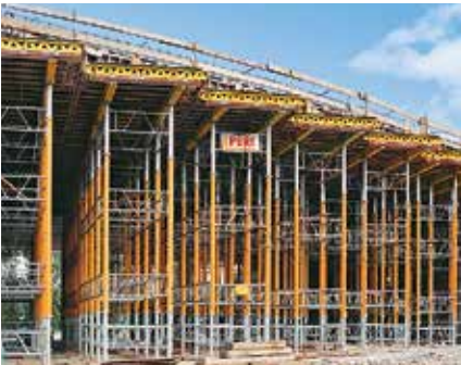
MULTIPROP Shoring Towers as sub-structures for project-specific slab tables.
