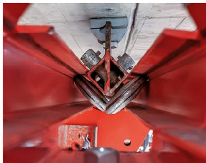
The VARIOKIT Cantilevered Parapet Track was suspended by means of rails and Roller Units from the underside of the bridge cantilever – at an identical position to the moving procedure and concreting.
