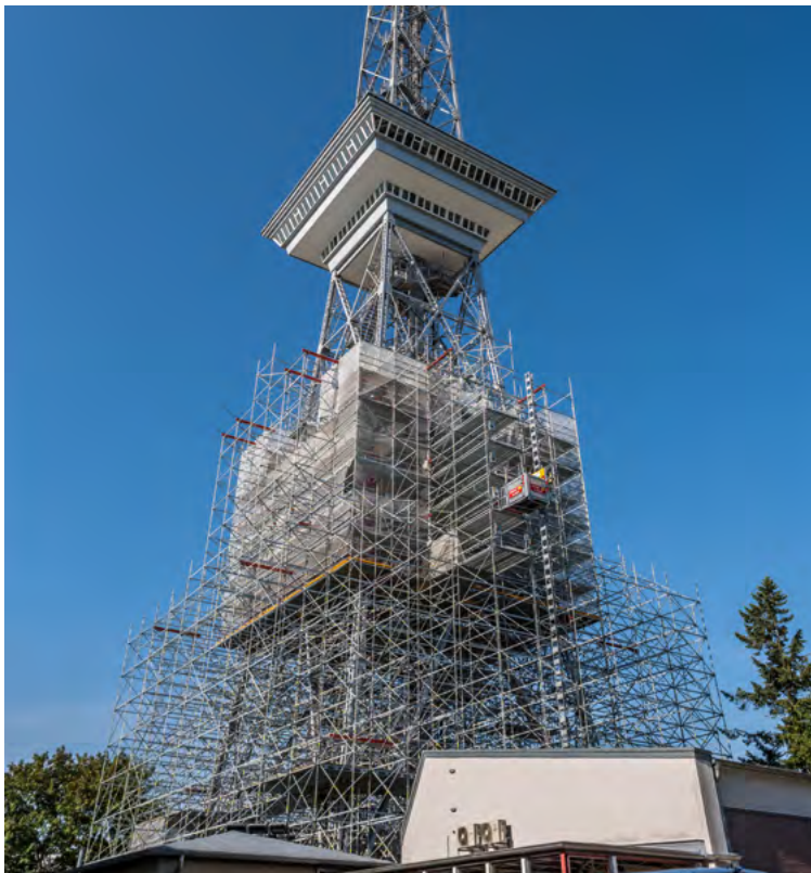
The old paintwork had to be removed and new corrosion prevention added, while the steel structure had to be completely re-painted.
