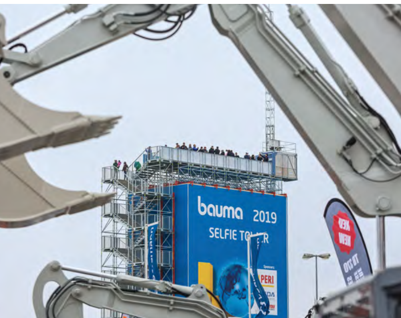
Use the exceptional construction techniques to your advantage to attract attention with your trade fair stands and exhibition areas.
