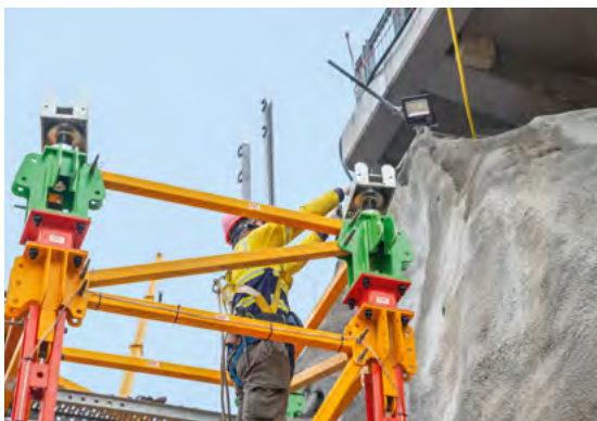
Height adjustments of +/- 75 mm are possible with the head spindle. What's more, you can adjust the head spindle by hand in an unloaded state. When under load, the Hydraulic Unit HD allows controlled lowering and lifting of the head spindle.
