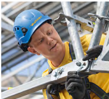
The ridge bars facilitate easy fixation of the roof inclination when lifting the LGS girder segments.
