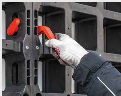
This connection allows you to position the panels in a flat and even manner. Once assembled, the couplers sit flush with the panel. This also allows
