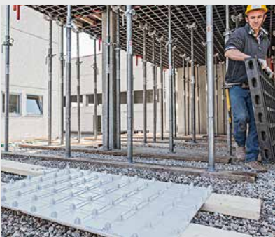
3. Installing the new formlining
