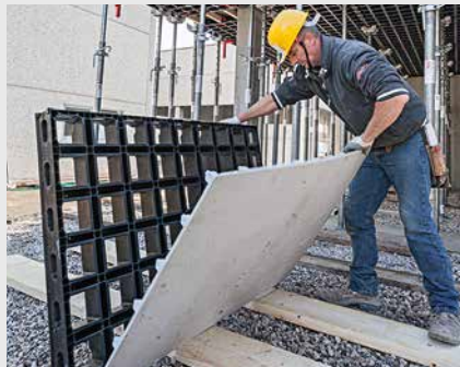
2. Removing the damaged formlining
