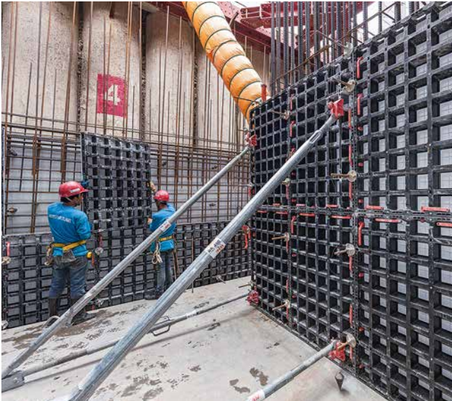
Low weight, small-format formwork elements – DUO showed off these advantages to the full with these basement walls.
