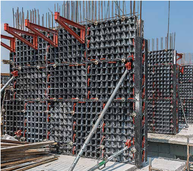
Successful first use of the lightweight universal formwork for the construction of shear walls.
