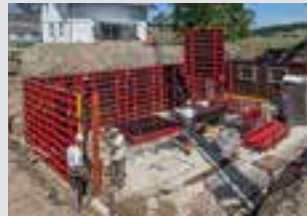
Wall Formwork
