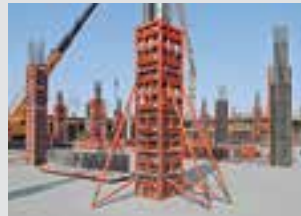
Column Formwork
