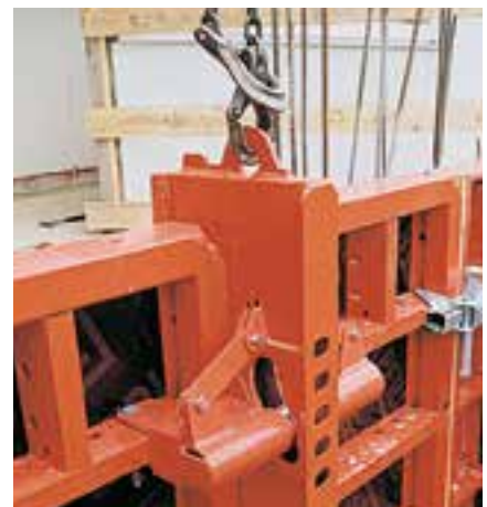
After being lifted by crane, the Shaft Panel TSE is released resulting in the required striking clearance.
