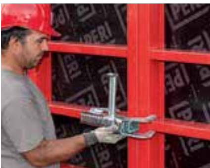
The BFD Alignment Coupler can be operated using one hand only.
