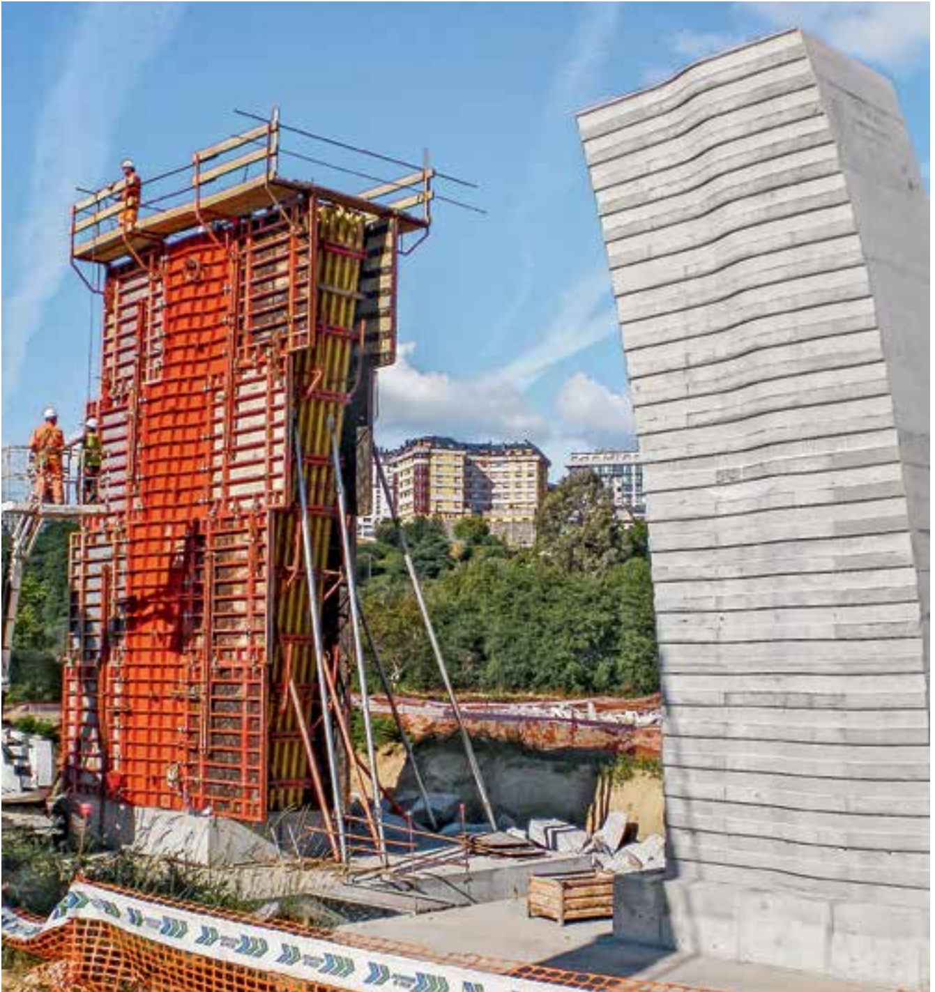
TRIO Structure being used to form a bridge pier: being covered with additional strips of wood results in an interesting surface structure.
