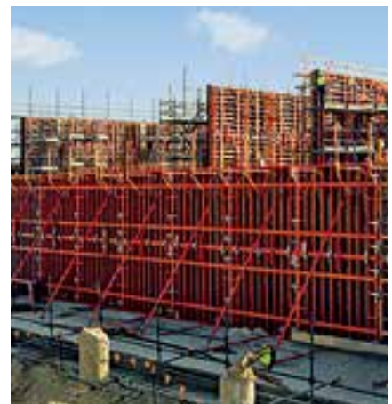
TRIO can be extended up to heights of 5.40 m in 30 cm increments. For larger heights, a compensation waler is also used.
