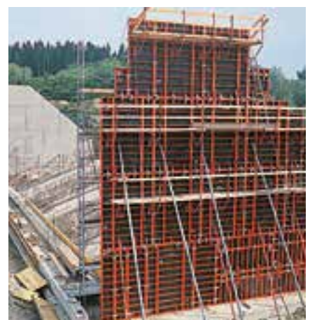
With TRIO 330, very high walls can be constructed very quickly – a 13.20 m high wall can be realized using only 4 panels.
