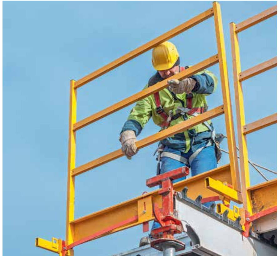
Side protection at cycle joints in the ground plan
