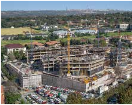
200,000 m 2 floor slabs brought into shape
