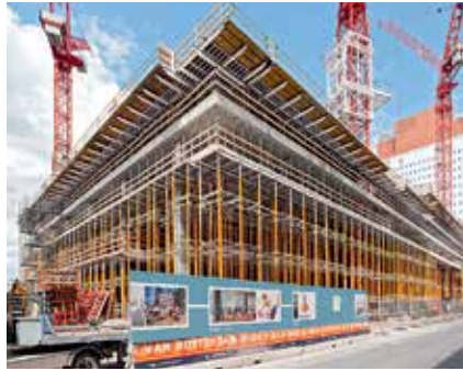
High level of safety at the slab edges
