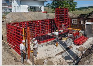
Wall Formwork
