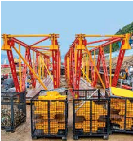
Pre-assembled girder packages can be temporarily stored on site using only a minimum of space until they are lifted to the next place of use.
