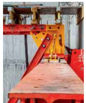
For high girder positions, without any possibility of positioning the towers, the Main Beam Bracket can also be used as a girder support.
