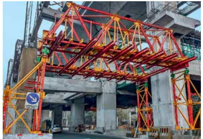
Elevated Metro Line, Hyderabad, India
