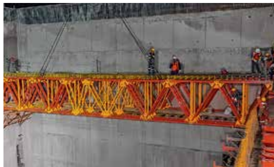
For high girder positions, without any possibility of positioning the towers, the Main Beam Bracket can also be used as a girder support.
