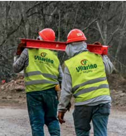
Handling the components requires a maximum of two workers.
