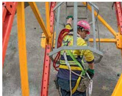
The ladder provides safe access to the Head Spindle Ring.
