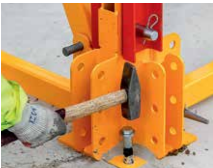
For anchoring the tower, the base point can be fixed in position with dowels.
