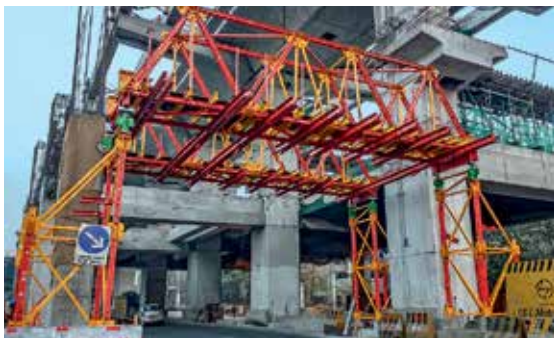
For a larger drive-through height, the Truss Girder can also be used horizontally at the top.
