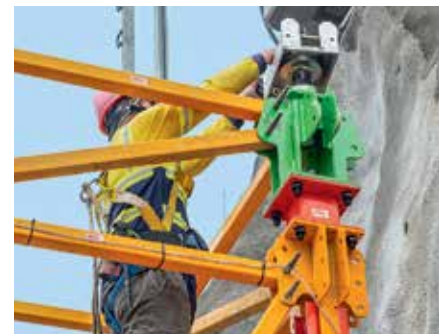
If the Head Spindle is not loaded, it can be adjusted by hand.
