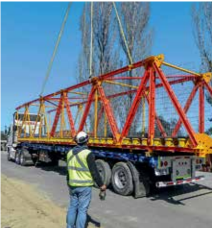
Pre-assembled units can be delivered directly to the construction site.
